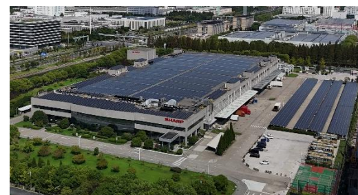
Solar Power Installation at our Manufacturing Facility in China
