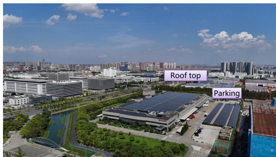
Solar power generation equipment
